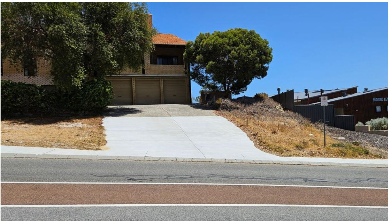
Figure 5: Existing northern crossover on Camberwarra Dr
