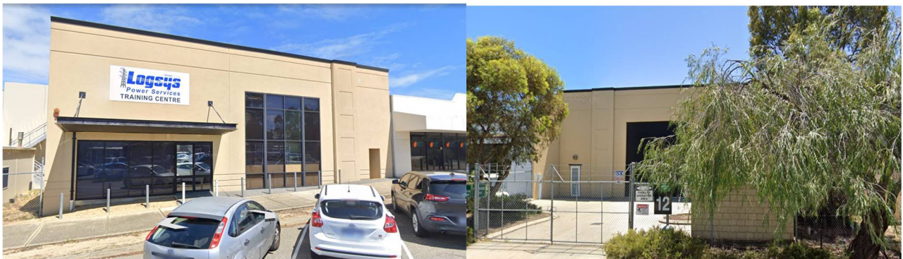
Figure 3 – The existing development on the subject land.
