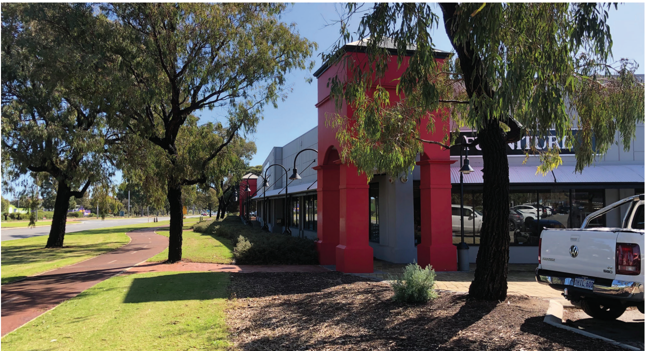
View of the existing western facade of the Harvey Norman Showroom
