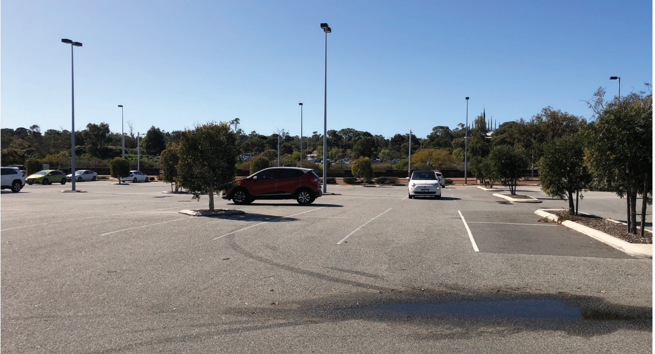
View of the existing at grade car park located in the southern part of the subject site
